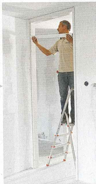
...the head and horizontal sections click into place...
