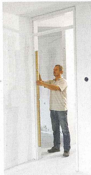
...a spirit level is used to check that the frame is straight...
