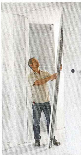
The vertical profiles are fitted onto the wall...
