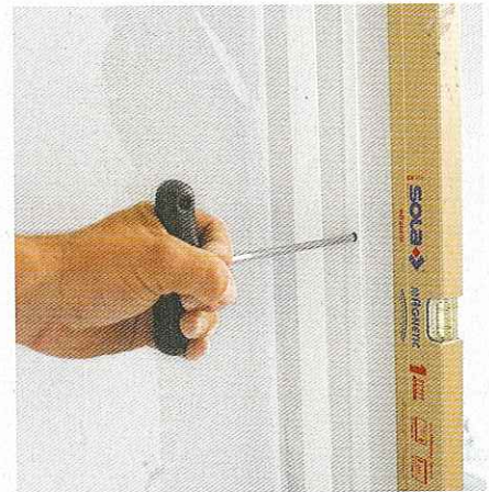
The profiles incorporate fixing holes to tighten the clamps.
